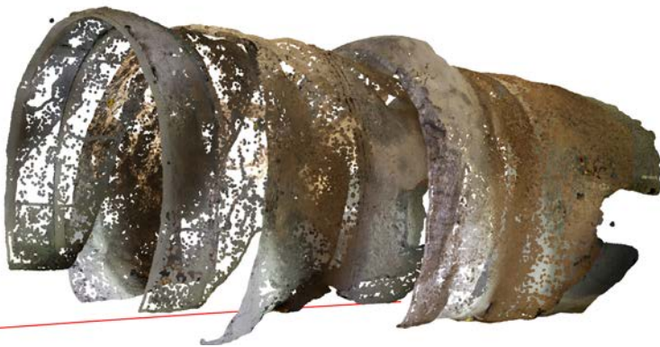
Control of tunnel trend
